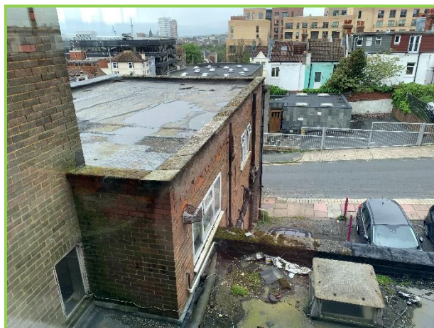
Poor flat roofing over flat and builder's workshop
